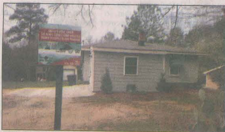
Lillie Mae Woods' 60-year-old home on Carrie Mae Lane in Stockbridge now has new life, thanks to upgrades funded through the Henry County Community Development Block Grant Home Owner Assistance Program.
